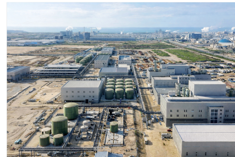
Aerial view of COBCO plant in Jorf Lasfar
