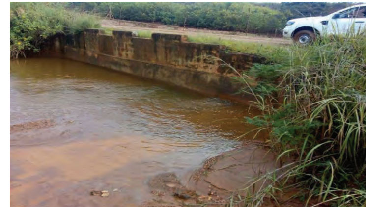
Figure 8: View of the position for the taking of sample 2 from the drain for the discharge of water from FQM's site.
